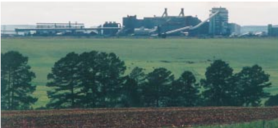
The Assmang ferrochrome facility about 8 km south west of Machadodorp, Mpumalanga, RSA. The 60 m-high building housing the new smelter may be seen on the right-hand of the picture.
